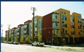
Emeryville CA Courtyards at 65th
