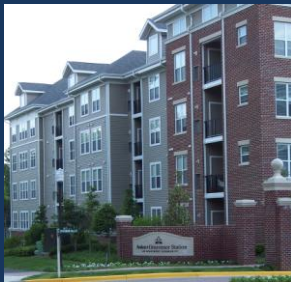
Montgomery County MD Grovesnor Station
